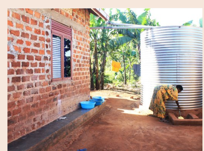
Water storage tank installed in a rural village in Uganda. http://water.org/post-p/catching-rain/
